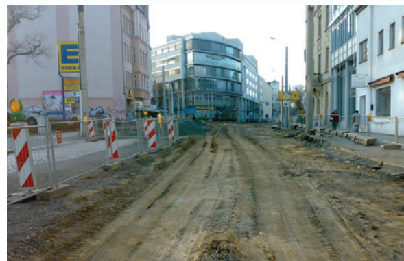
ROAD CONSTRUCTION IN PLAUE 2009
